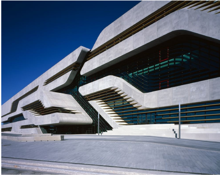
Over 1,000 concrete panels comprise the facades of pierre schlegel Photo: Hélène Binet
